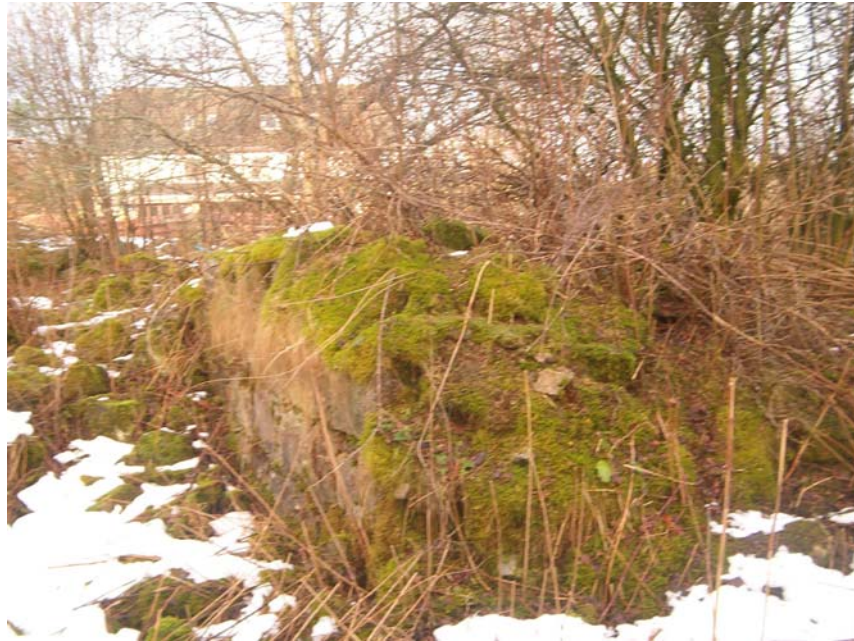
Fig 8. Showing remains of Mill
